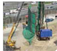
Installing Temporary Soundproof Barriers
